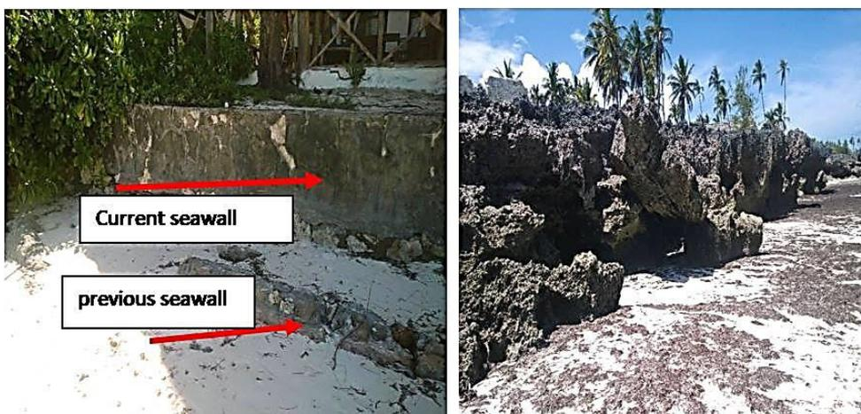
**Figure 12: shoreline erosion where new seawall is built inward compared to the former at Pwanimchangani (left) and cliffs fall due to wave erosion at Matemwe (right)**
