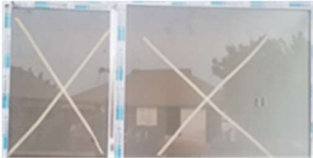
Figure 3: Sign X Indicating Unfinished Work in Kigamboni, Dar es Salaam (2022)
