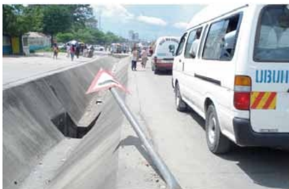
Figure 4: Knocked “Speed Hump” warning sign (Morogoro road – 565 m from Ubungo traffic light)
