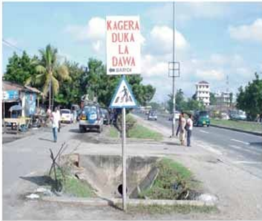
Figure 6: Advertisement placed on top of the sign and worn out pedestrian zebra crossing (Morogoro road – Kagera Area)
