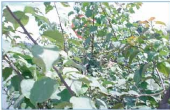
Figure 2: “No U Turn” Regulatory sign hidden by vegetations (Ubungo area, 255 m from Ubungo Traffic lights)
