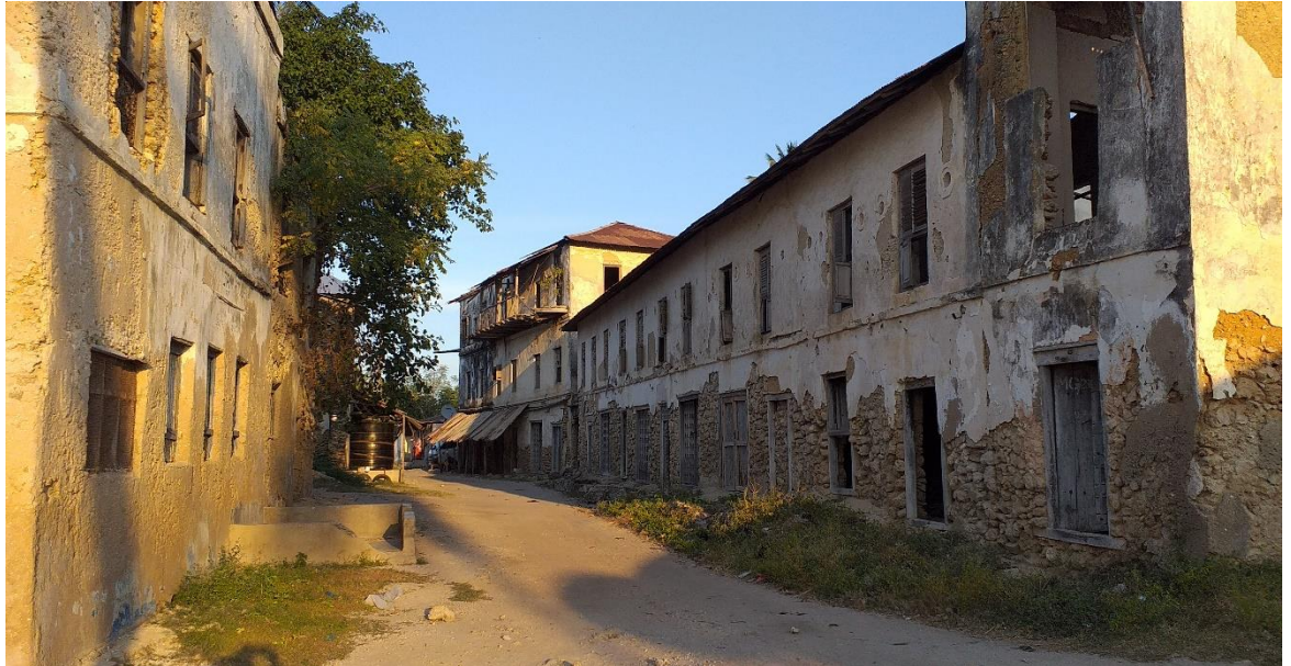
Figure 2: A section view of Indian Street at Kilwa Kivinje. Author's photo, 2018
